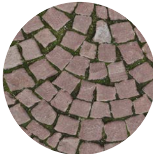
Permeable Paving for Stormwater
